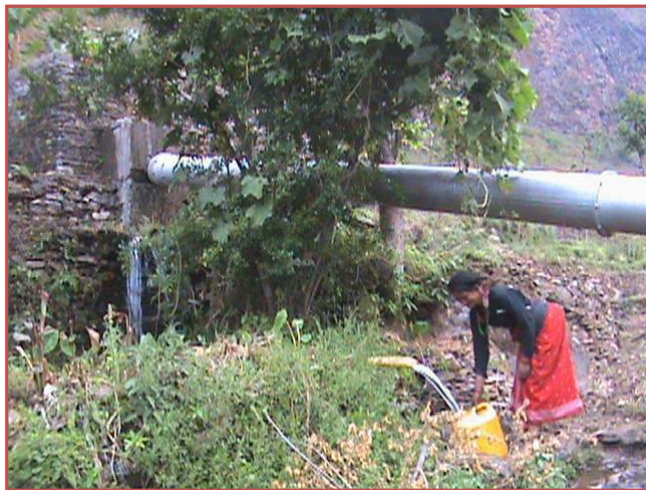
Figure 28: A women collecting water that is leaking from the Forebay tank of Kailashkhola-IV MHP
