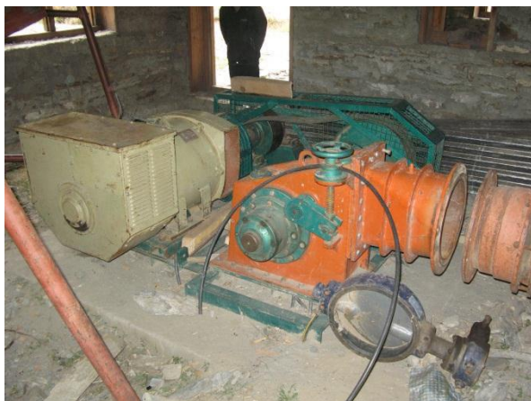
Figure 40: Turbine and generators in Powerhouse of Kukrfalna MHP
