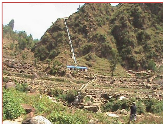
Figure 21: General view of Kasegad MHP ( forebay, penstock pipe, powerhouse and tail-race)
