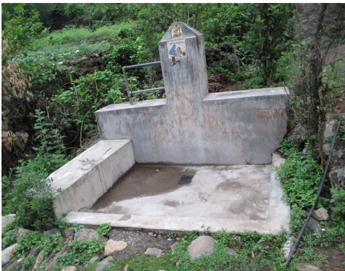
Figure 2: Non-functional tapstand of NEWAH supported scheme in Dhuligada VDC
