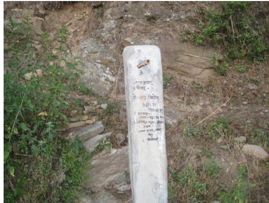
Figure 20: A non-functioning tapstand
