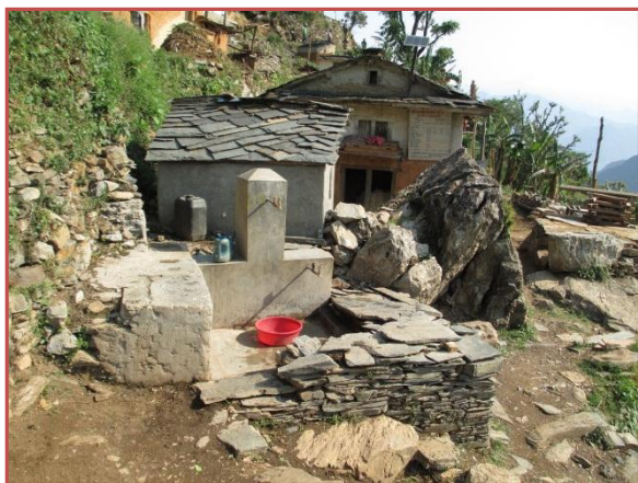
Figure 25: Tapstand protected by stones to prevent damage from live stocks
