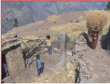
Figure 22: Non-functioning tapstand in Bishal Bazar Dalit village
