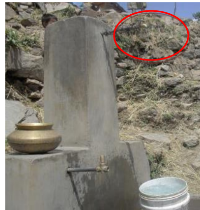
Figure 10: A tapstand with broken child tap. Tap for adults (seen above) is protected by barbed wire so that children cannot use the tapstand
